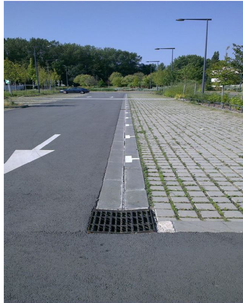
The image above shows semi-permeable pavers and underground detention systems designed to provide both parking and storm-water management.
